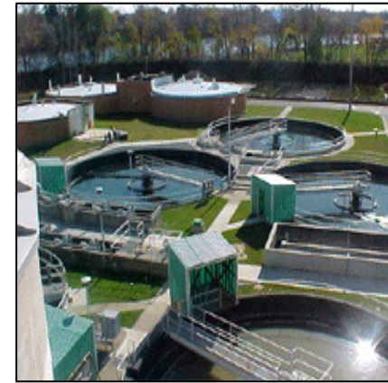
Water Treatment Plants
